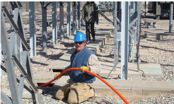
FIGURE 4: Fibre optic cable installed in substation yard.
