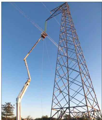
Fig. 5: The robotic arm in use during the restoration.
