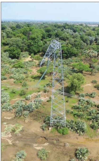
Fig. 1: Damaged towers which had to be repaired.
