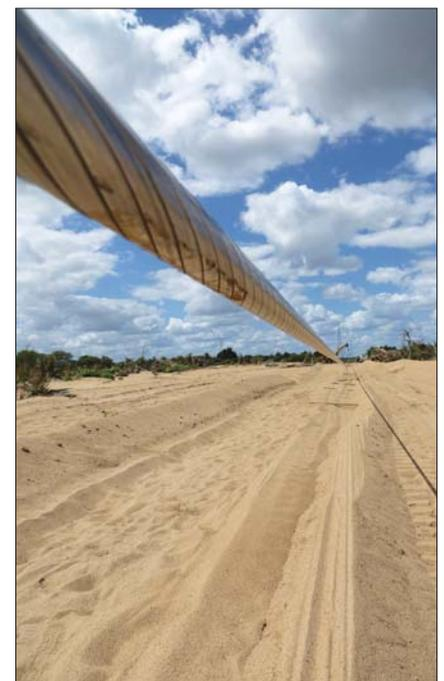
Fig. 3: ACCC Lisbon conductor was used in the repair of the section.
