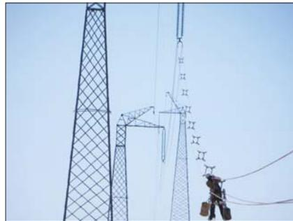
Fig. 2: Fitting spacers on the new section.
