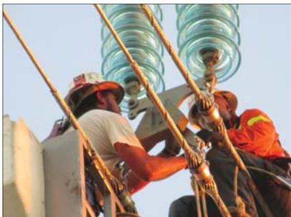
Fig. 4 : Using ACDC conductors made it possible to utilise a three-bundle configuration.
