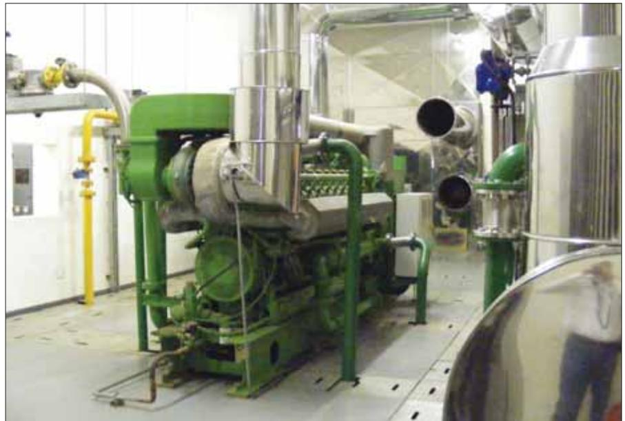
Fig. 1: MTN Campus GEJ320 engine/genset trigeneration unit being installed.
